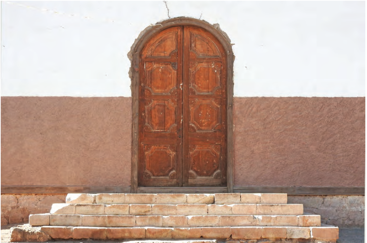
Puerta principal con escalinata de piedra | Main entrance with stone perron
