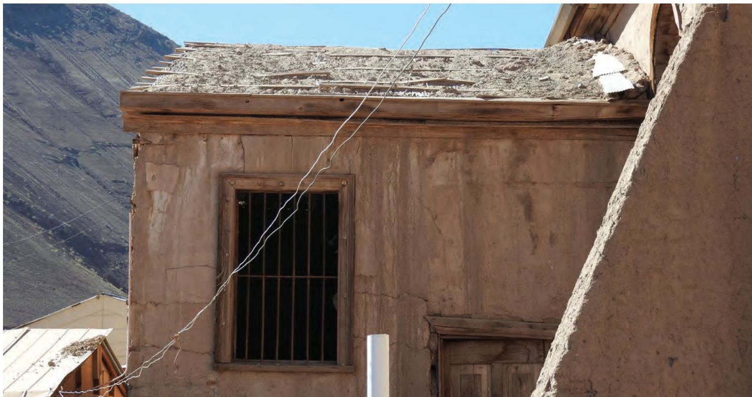
Bodega | Storage room
