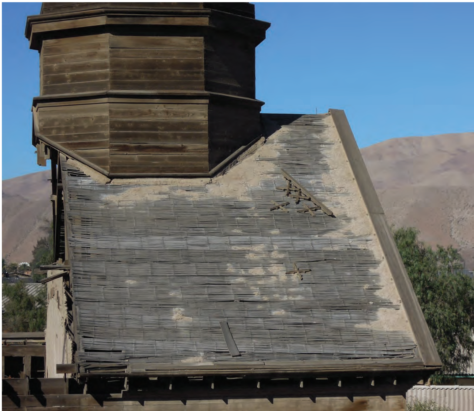
Techo original con restos de la cubierta de barro | Original roof covering with rests of the loam cover
