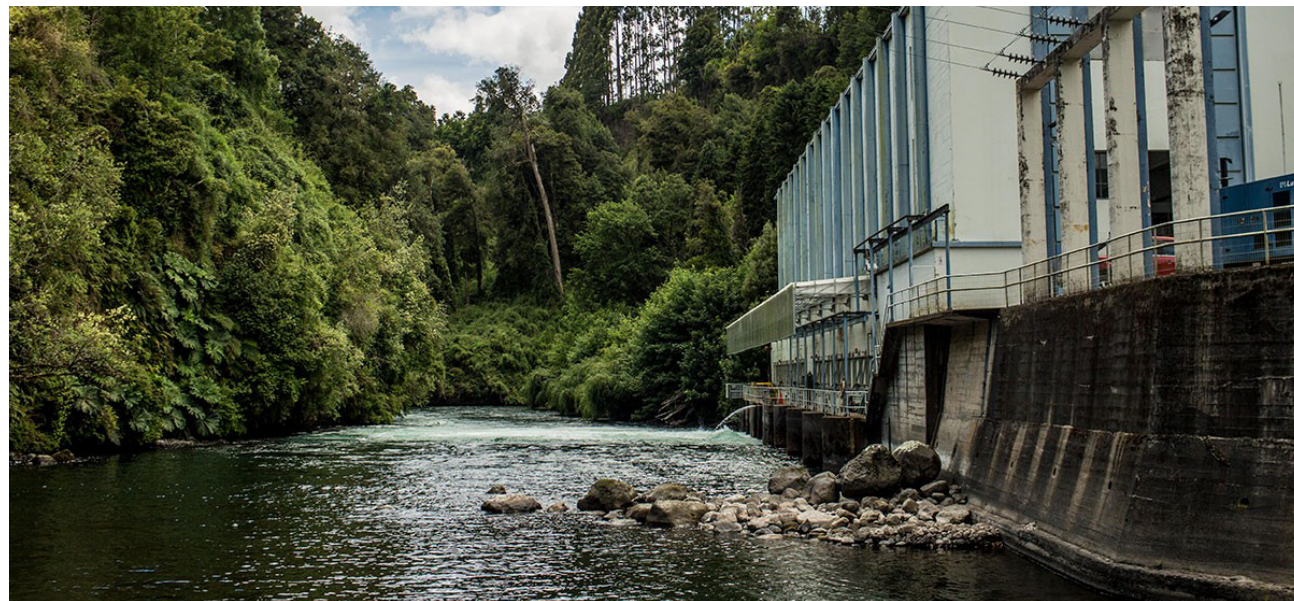
Pilmaiquén hydroelectric power plant. Enel (Chile).
