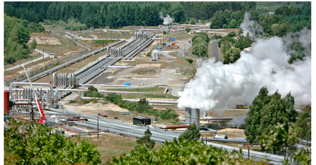
Wairakei geothermal power plant, New Zealand.
