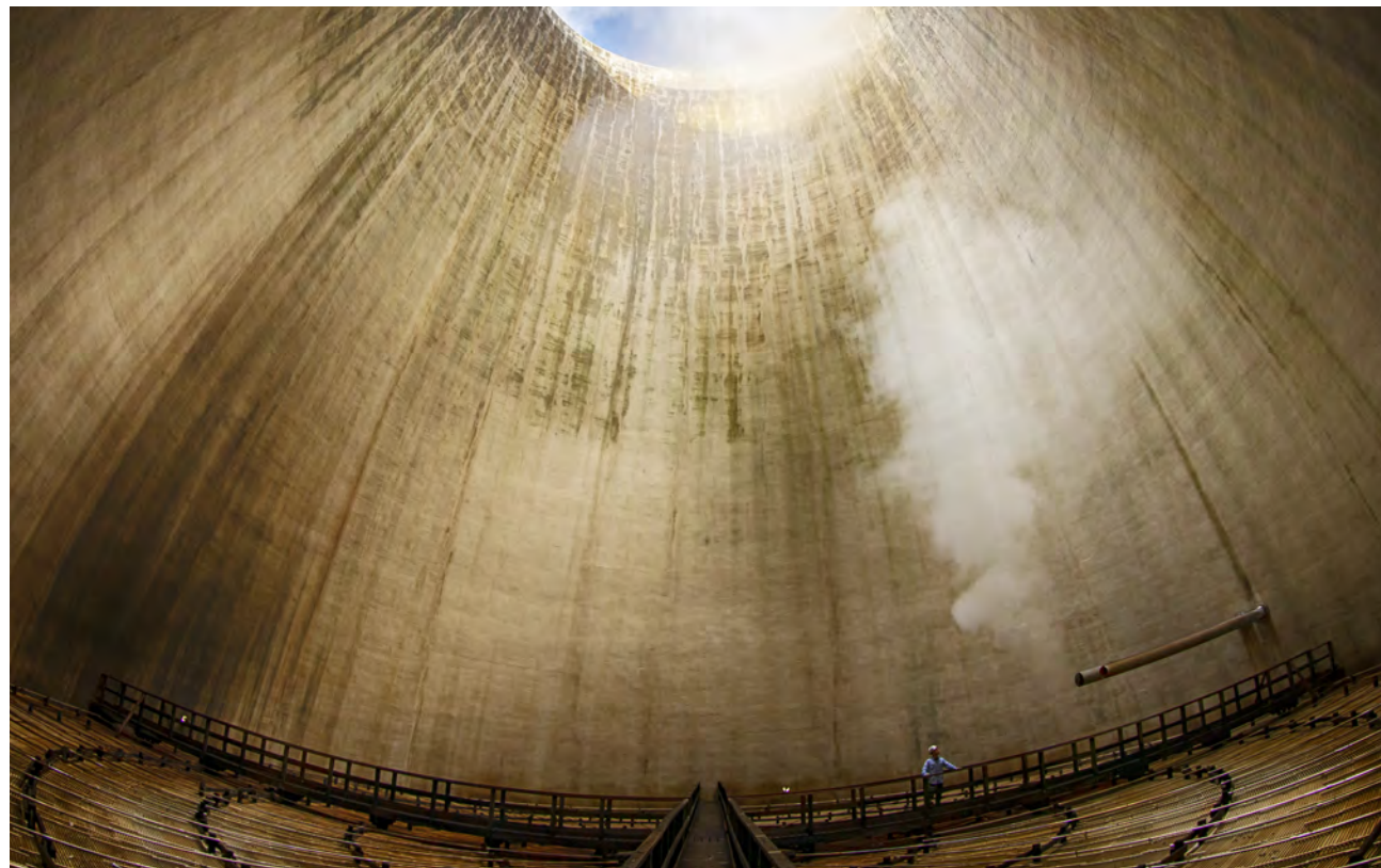
Interior of a cooling tower at Larderello. Its dimensions can be better appreciated by looking at the human figure at the bottom. Fabio Sartori Collection (Italy).
