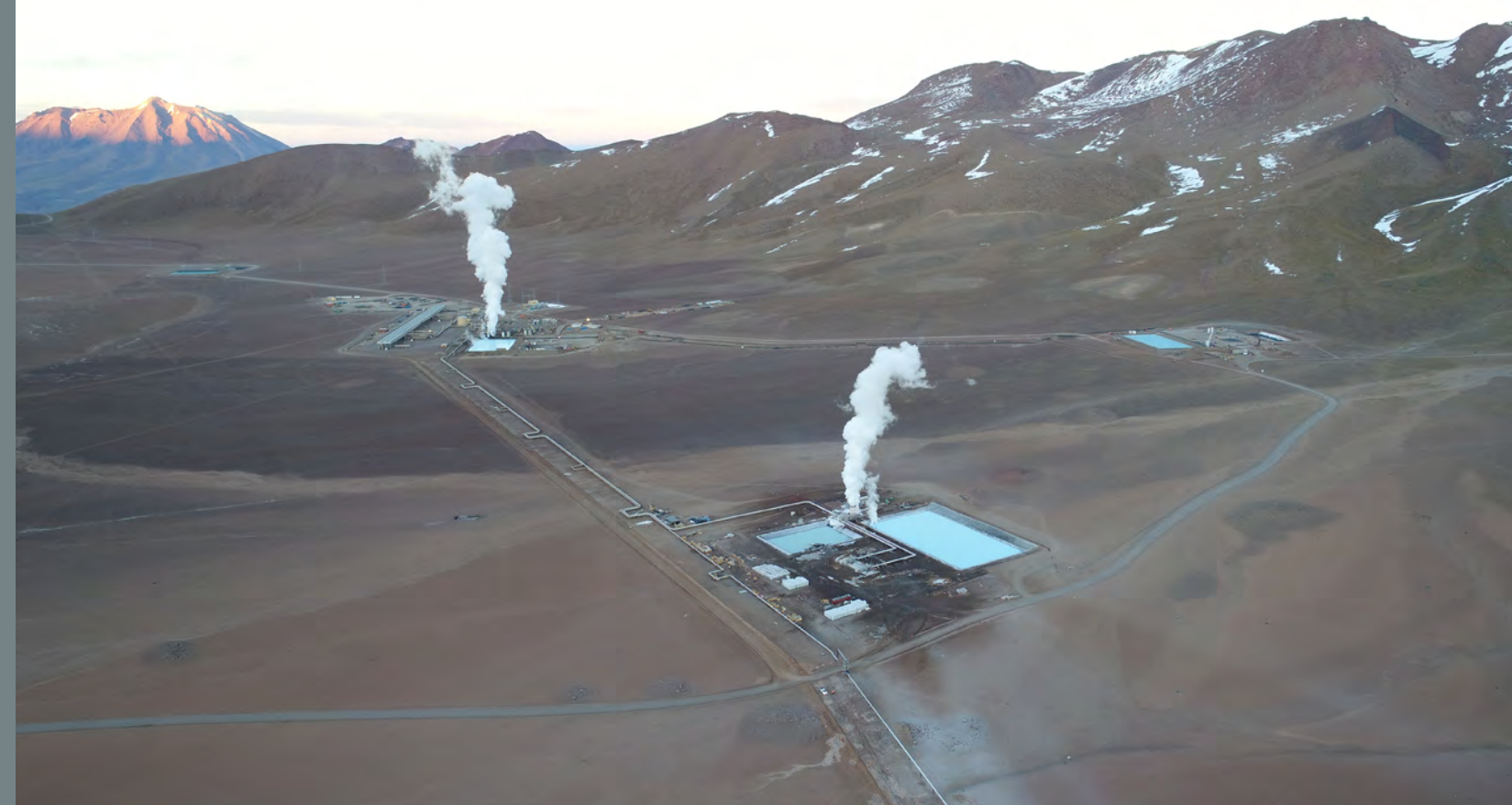
Geothermal energy is already making an important contribution to the decarbonization of the Chilean energy matrix. Enel (Chile).
