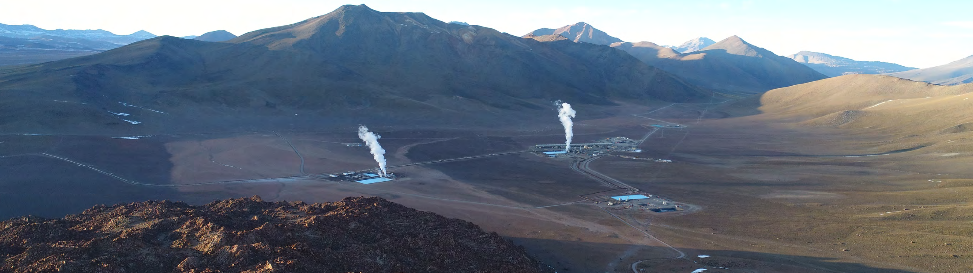
Panoramic view of the sector where the only geothermal power plant in South America is located. Enel (Chile).
