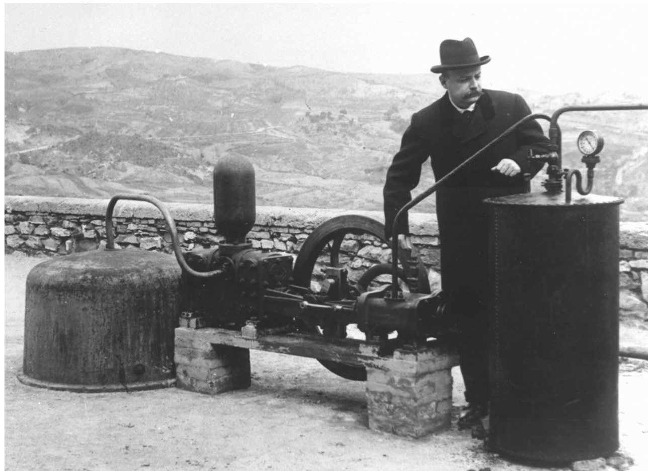
Technological leap. In 1904, Piero GinoriConti produces for the first time electricity based on geothermal energy. Enel Historical Archive (Italy).
